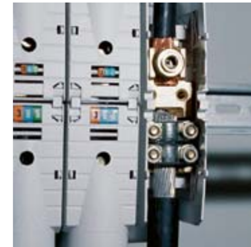
< Alumin./copper direct connection
