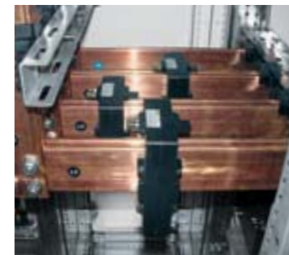
^ Fixing CTs on busbars
