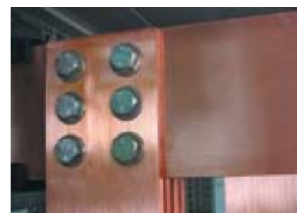
^ Connection on 120 x 10 bars (4000 A)
