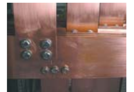
^ Double connection: 100 x 10 bars (3200 A) and 80 x 10 bars (2500 A) on common 120 x 10 bars
