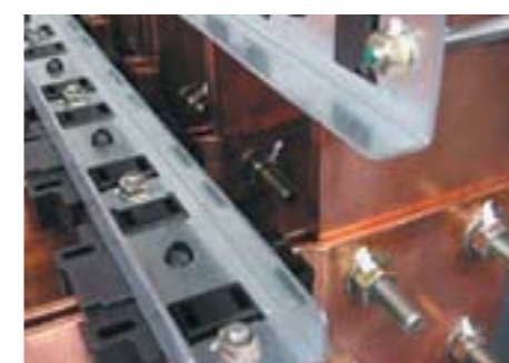
^ Connection on 120 x 10 bars (4000 A)
