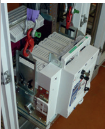
Installing a draw-out DMX 3 in its base
