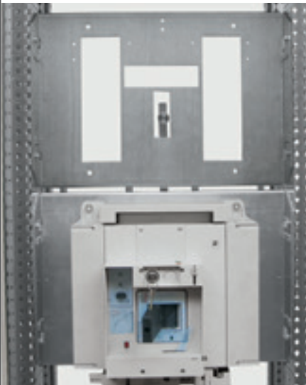
DPX 3 1600 supply inverter being mounted
