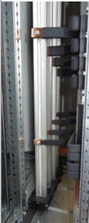
Busbar installed in cable sleeve.
