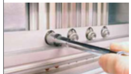
The row distribution blocks are pre-equipped with hammer head bolts. Tighten them to connect the block to the busbar.
