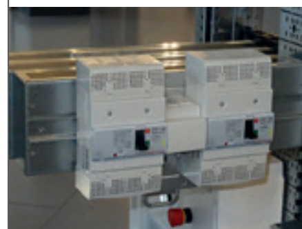
2 - Clipping the rail onto the attachment pieces (2 positions)
