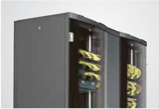
LCS 2 enclosure with integrated cabling unit
