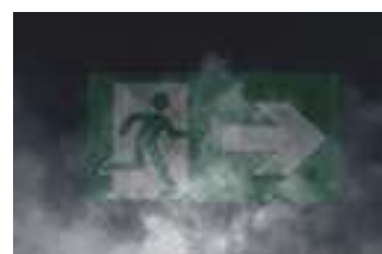
Badly illuminated exit sign
