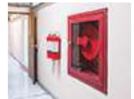
Near each place of fire-fighting equipment
