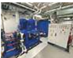
Plant rooms for generators and control equipment
