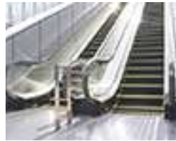
Escalators to enable users to safety disembar
