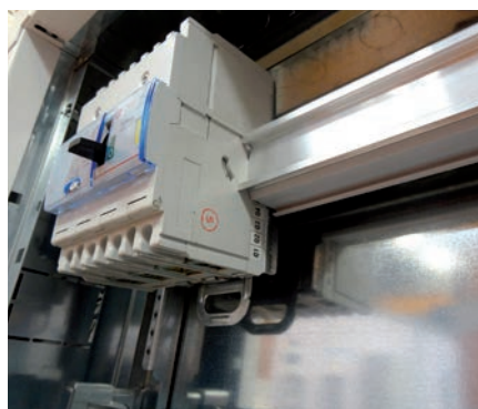
Installation of a plate + MCCB on the rail.
